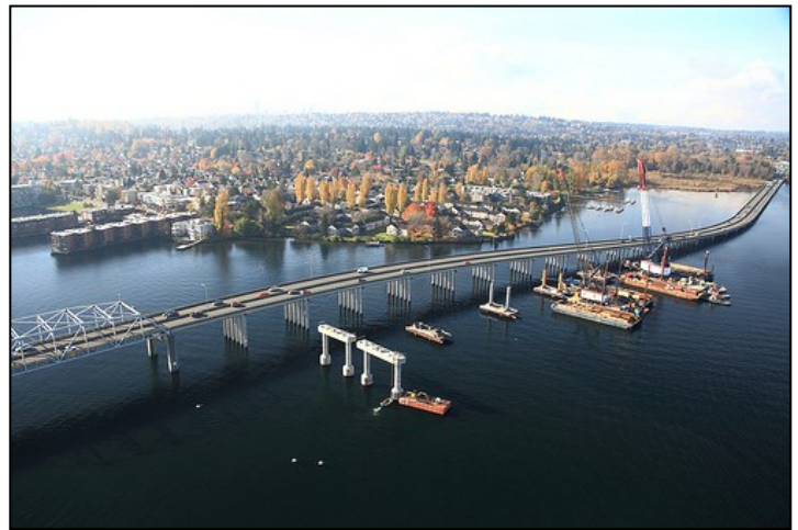
SR 520 Floating Bridge and Landings Anchor Design
