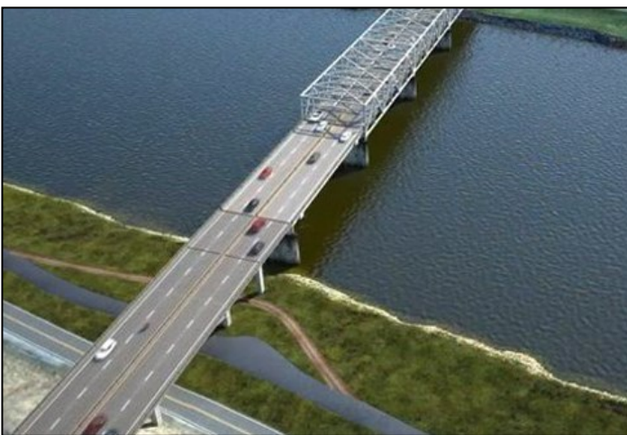
I-5 Skagit River Bridge Replacement
