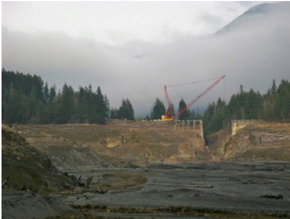
Elwah Dam coming down!
