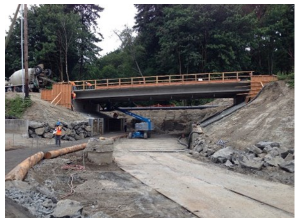
Bridge and path (at left)
