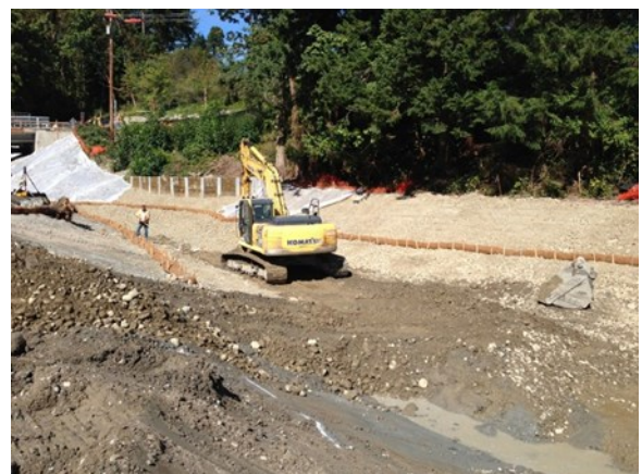
Excavating new stream channel
