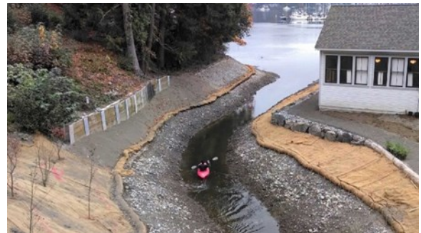
Channel near completion
