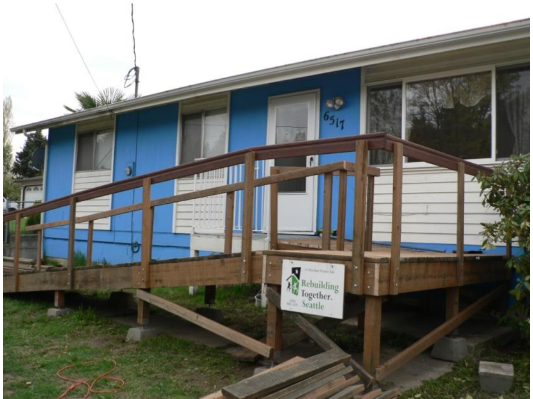
Last year's project added access ramps to this house, along with painting and flooring improvements and other small projects.
